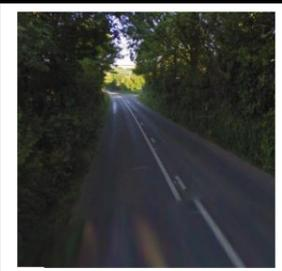
Dragons teeth to be installed before the left hand corner leading into the village. **SINGLE HEIGHT** Standard CC spec dragons teeth ending prior to junction. Min 150mm spacing from double white lines to avoid visual bleeding of lining.
